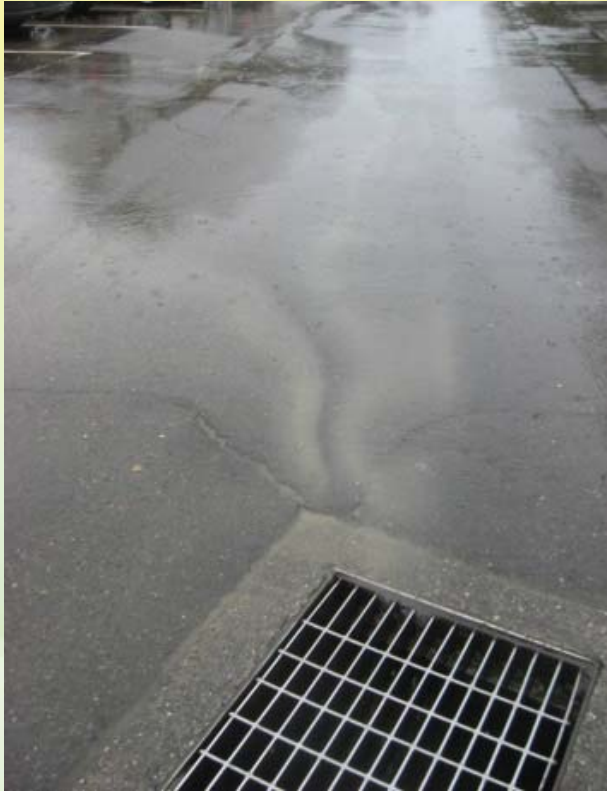
Drain Inlet - Campus
