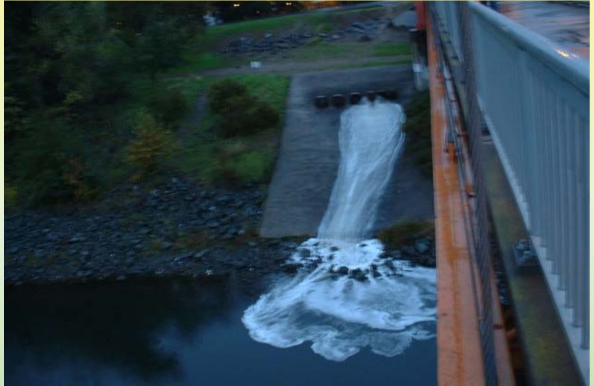
Storm Drain Discharges into American River
