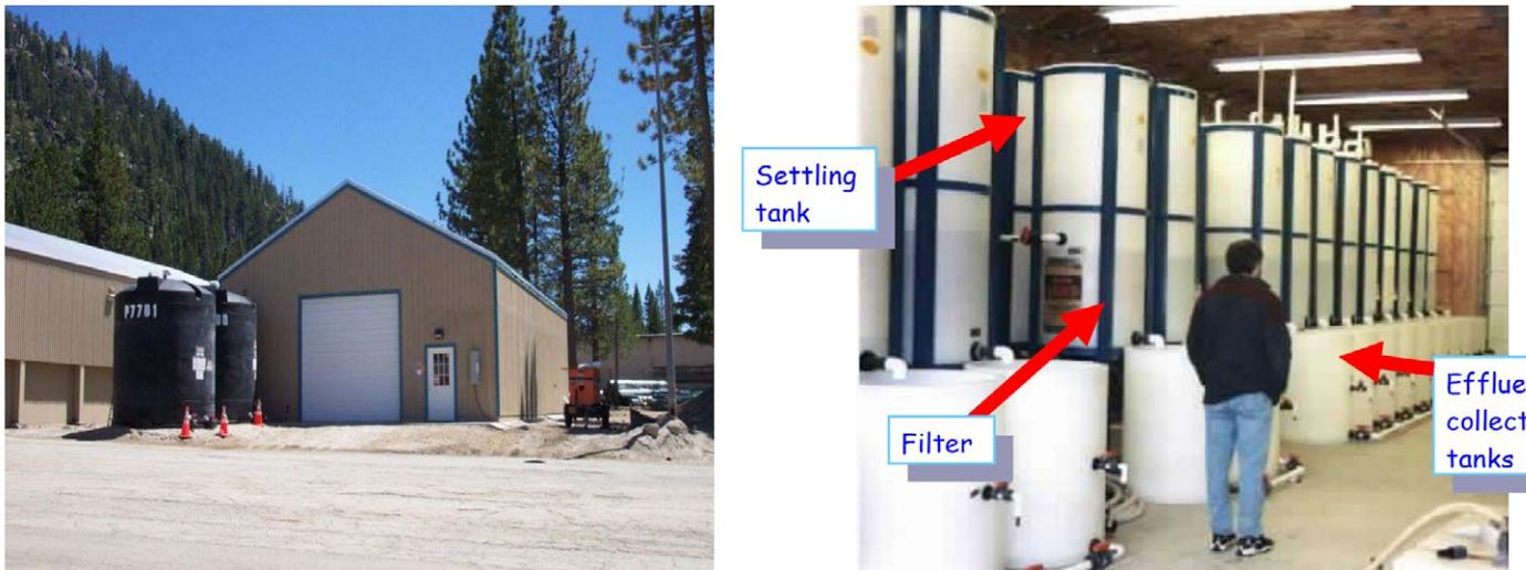
**Figure 1 Photographs showing (a) pilot treatment building with storage tanks, and (b) sedimentation and filtration units**
