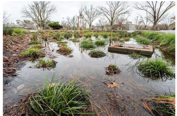
Bioretention planters are a part of the network of stormwater management devices used to store rainwater and filter runoff that flows into the nearby American River. (Sacramento State/Morgan Murphy)
